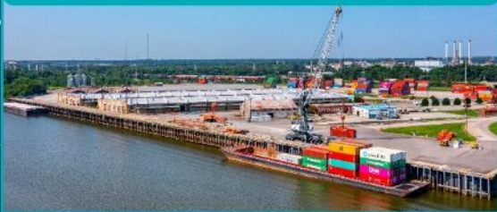
RICHMOND MARINE TERMINAL
